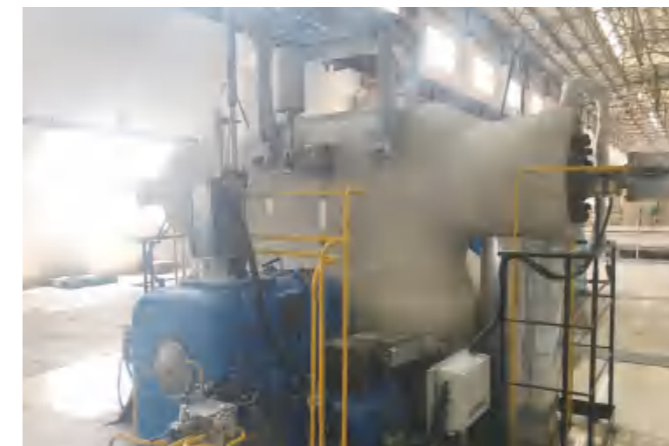
◆ 南通江山农药化工股份有限公司 12MW背压汽轮机 Nantong Jiangshan Agrochemical & Chemical 12MW Back-pressure Steam Turbine Unit
