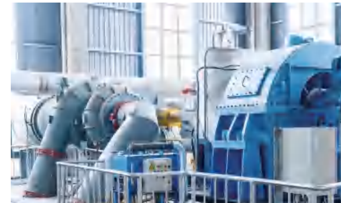
安徽丰原集团年产15.36亿方汽轮机拖动空气压缩机 Anhui Fengyuan Annual Output of 1.536 Billion m 3 Steam Turbine driven Air Compressor
