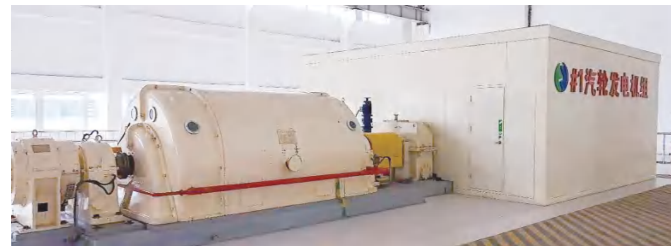
◆ 沈阳西部环境垃圾焚烧发电项目汽轮机组 Shenyang Waste Incineration Power Plant Steam Turbine Unit
