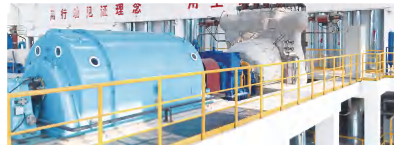
◆ 山西高义钢铁15MW发电项目汽轮机组 Shanxi Gaoyi Steel 15MW Power Generation Project Steam Turbine Unit
