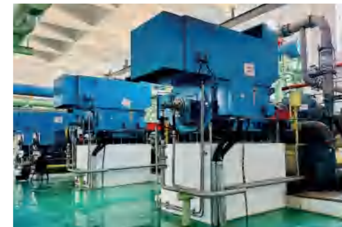
◆ 南通天生港发电厂汽拖空压机集中空压站项目 Nantong Tiansheng Port Power Plant Gas-driven Compressor
